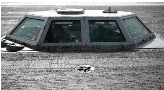
▲ CATAPULT CONTROL POD This observation pod, which retracts below the flight deck, enables the crew controlling catapult launches to see what's happening while remaining safe from moving aircraft.
